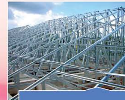
Steel Roof Truss
