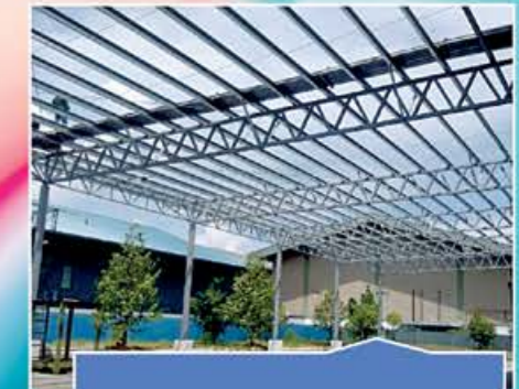
Mild Steel Structure
